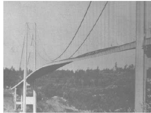
Figure 4 - Takoma bridge failure (1940)
